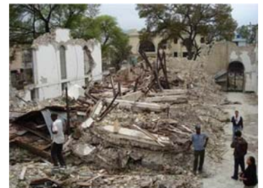
St. Trinity Episcopal Cathedral collapsed building and site, Port-au-Prince. Photograph by Corine Wegener.
